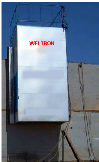
Overall view of system
