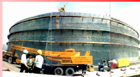
WGW 3M in operation
